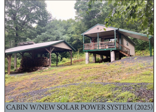
CABIN W/NEW SOLAR POWER SYSTEM (2025)
