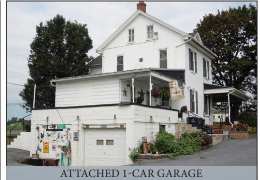
ATTACHED 1-CAR GARAGE
